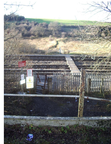
An access point to the The Carrs LNR at Ferryhill
